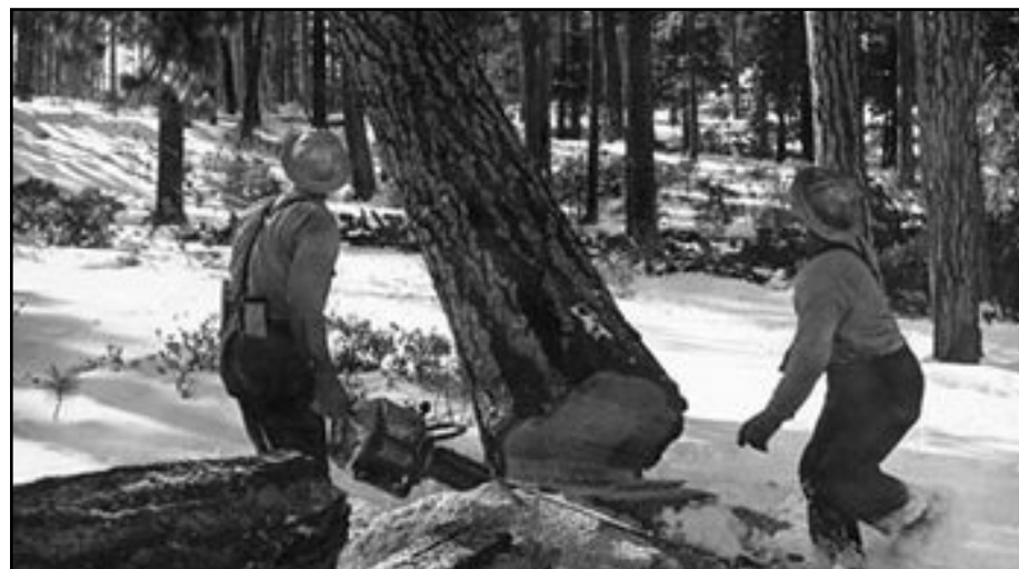
Chainsaws in the Cathedral
